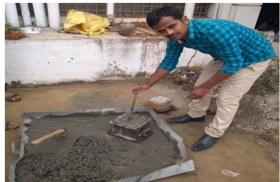
Fig. 2: Placing & compacting of concrete
